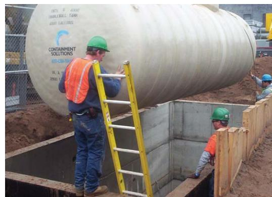
Workers install piping and product storage tanks as part of the 10 new dual-pump recovery wells at ExxonMobil's Greenpoint Remediation Project site. All wells are expected to be fully operational by the end of the year.
